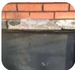
Lintels rebuilt with 571 Concrete Repair LW
