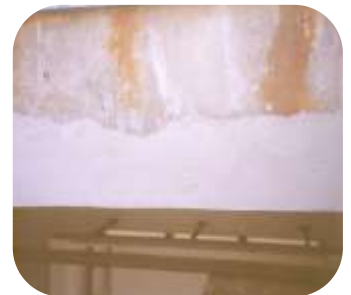
Overhead concrete surface rebuilt with 571 Concrete Repair LW
