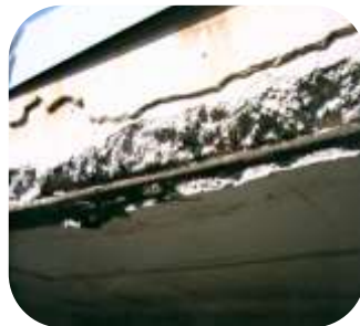
Overhead concrete surface rebuilt with 571 Concrete Repair LW
