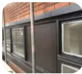
Lintels rebuilt with 571 Concrete Repair LW
