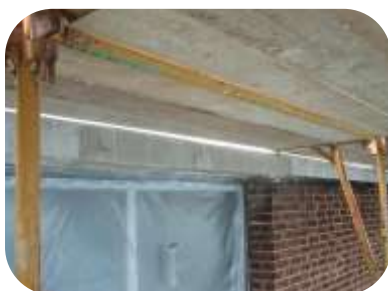
Damaged lintel rebuilt with 571 Concrete Repair LW
