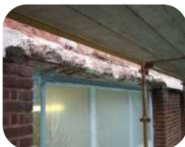
Damaged lintel rebuilt with 571 Concrete Repair LW
