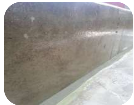
Concrete wall suffering from weather and UV degradation sealed with Resichem 505 Damp Seal
